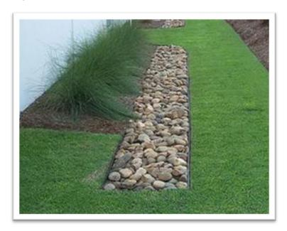
Before beginning, determine the soil type in the location where you would like to dig your trench. An easy way to do this is with the ribbon test (see page 8). If you have clay soil, the drainage will be poor. In this case, a vented pipe can be added amidst the gravel to let water flow through the pipe to a lower/better-draining area of the property.
